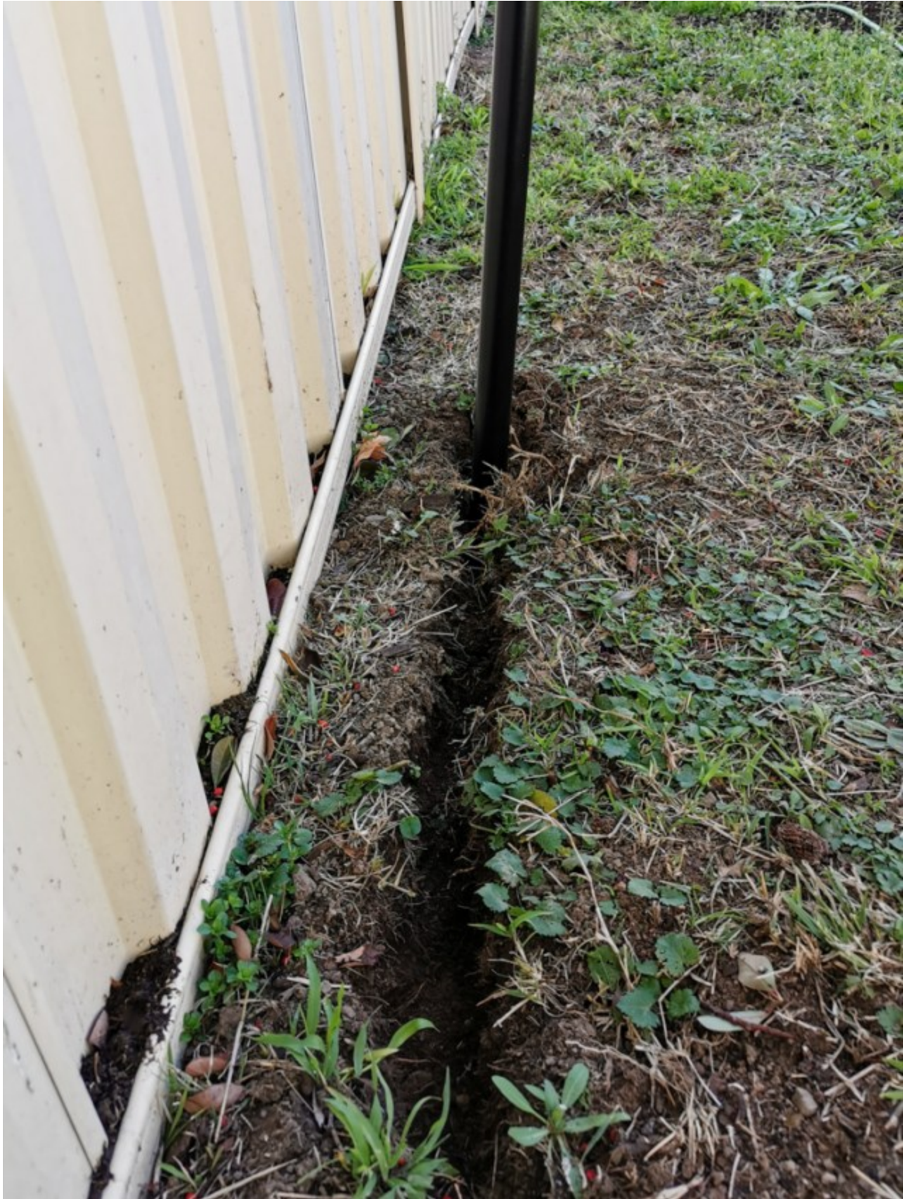
Root barrier trench cut using Slammer Tool, no digging required!
