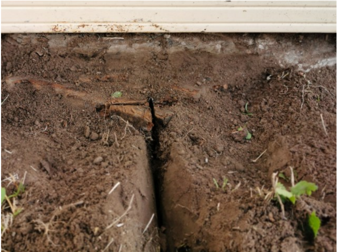
Slammer Tool cut through tree roots and compacted soil filled with stones
