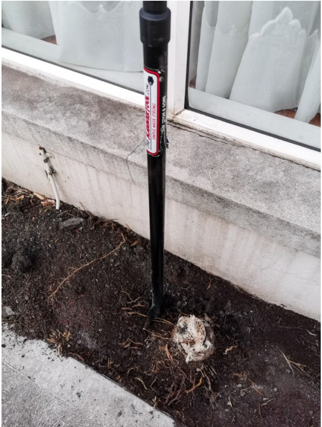
Slammer Tool cutting out broken yucca stump
